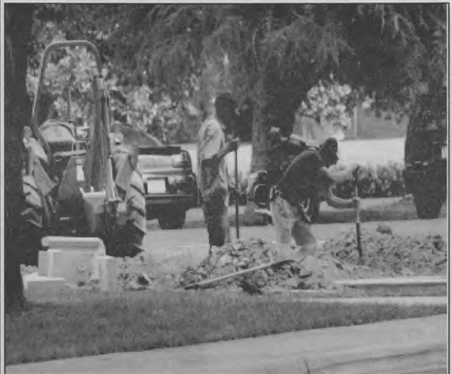
Construction continues throughout campus... President Nido Qubein unveiled the plans for the next three years at a special assembly of students, faculty, and the High Point community at large on Sept. 13.
